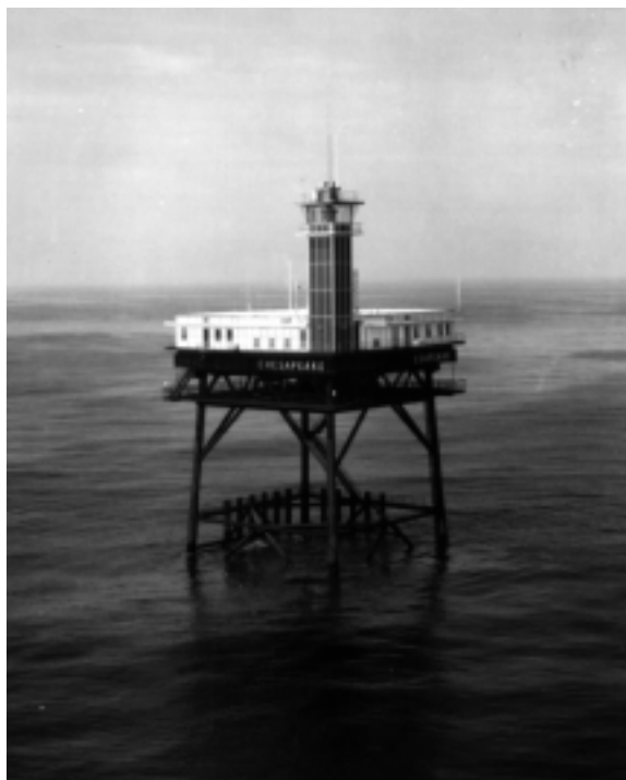
Figure 9. Chesapeake Light Station, Texas tower at entrance to Chesapeake Bay.
