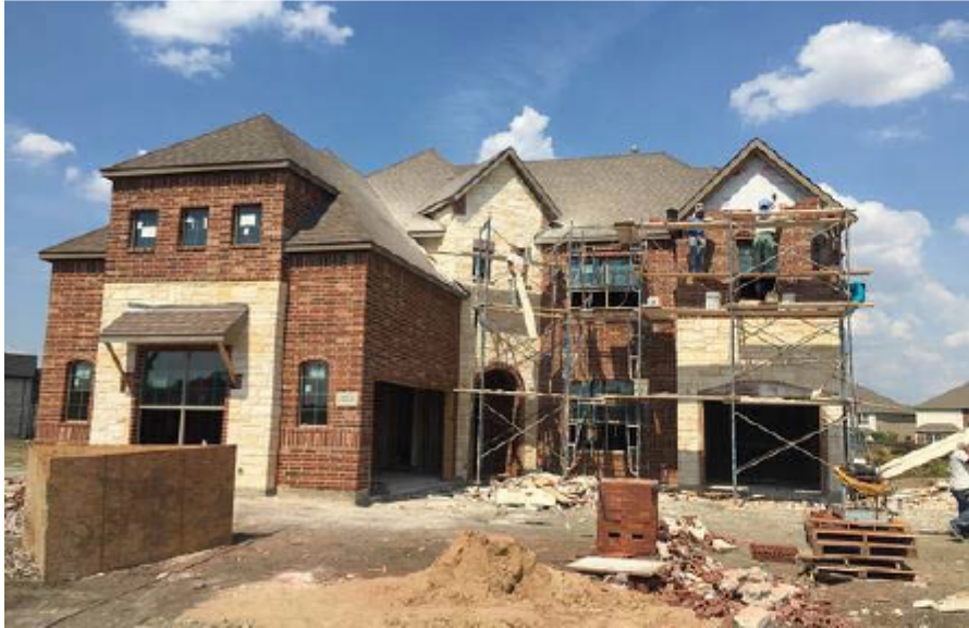
Crews construct a Ryland Group home near Dallas.
