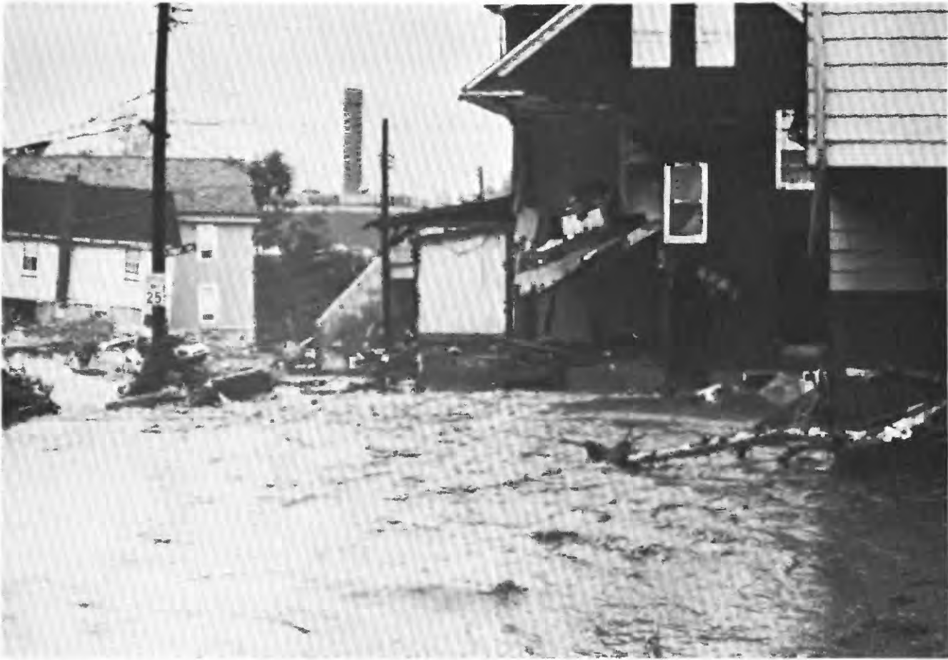
FIGURE 33.—Home damaged by flooding from Solomon Run in the Walnut Grove section of Johnstown (Johnstown Tribune-Democrat photograph.)
