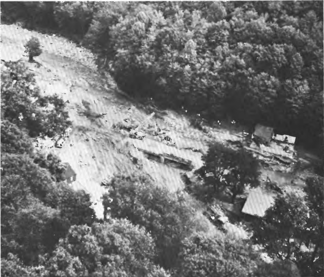
FIGURE 31.—Flood damage downstream from the Laurel Run Dam. The foundations of two homes that were washed away are visible in the upper left corner (Pennsylvania Air National Guard photograph).
