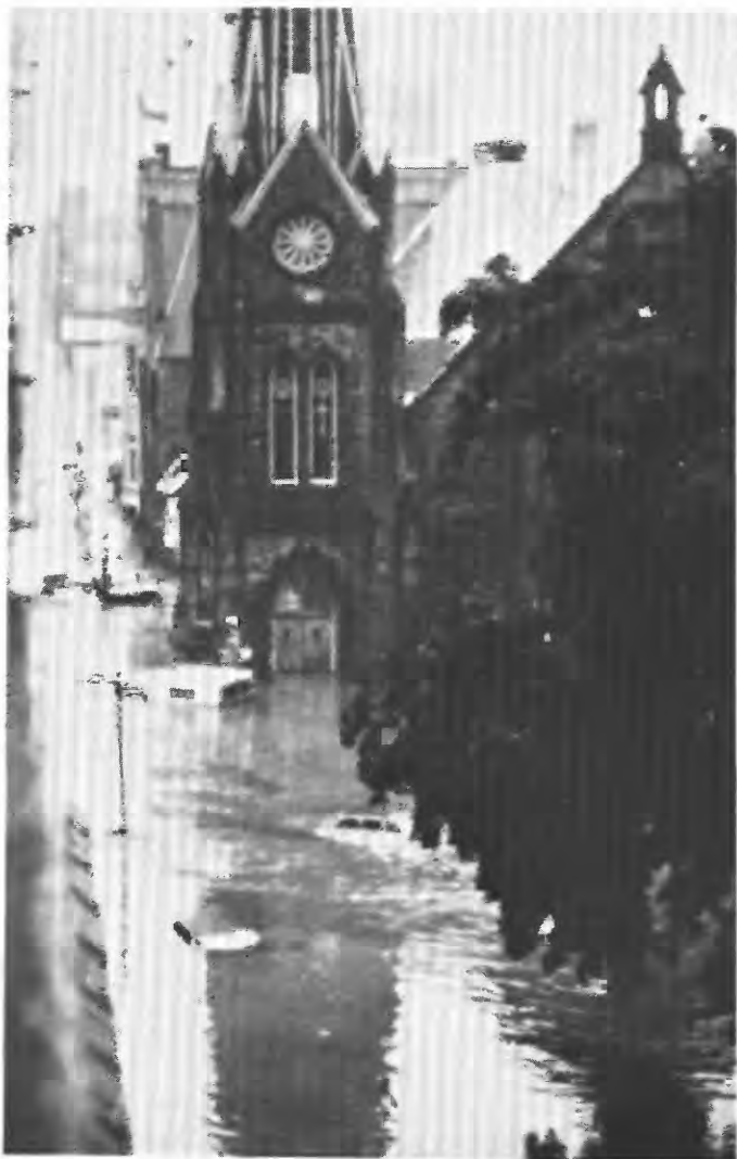
FIGURE 22. - Flooding at Franklin Street United Methodist Church in Johnstown. (Johnstown Tribune-Democrat photograph.)
