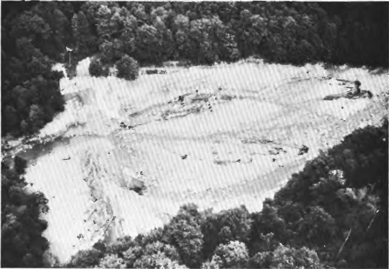
FIGURE 19.—Aerial view of breach in Sandy Run Dam (Pennsylvania Air National Guard photograph.)
